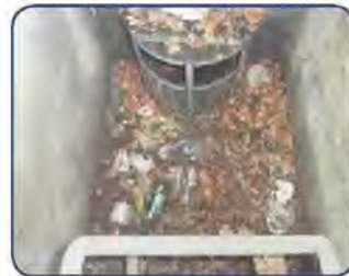
The City cleans and inspects 250 trash capture devices quarterly, removing 40 cubic yards of debris annually.
