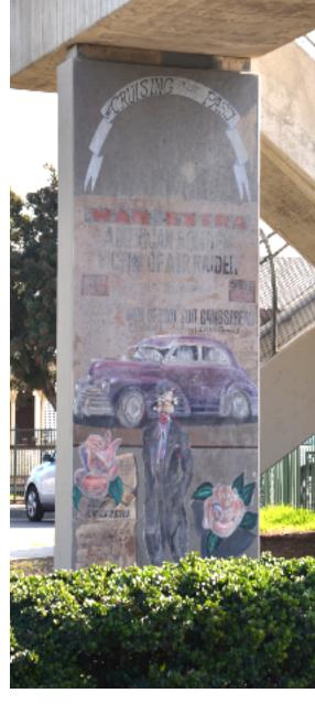
• Apply acrylic polymer coating, with a second coat of two-part Permashield premium protective coating that is anti-graffiti and protects from UV rays.
