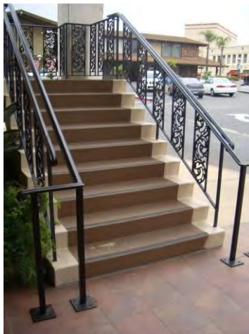
New ADA, stair nosing and handrails
