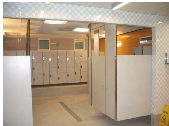
New Dressing Stalls and Floor Drains
