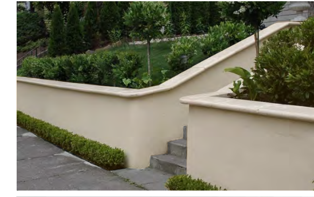
(N) Stucco Retaining Wall
