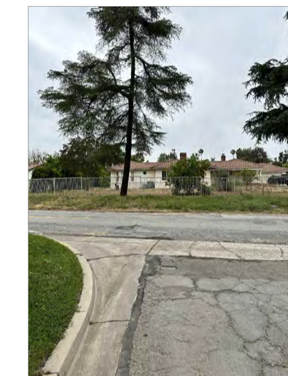
11. EXISTING BUILDING ON SITE
