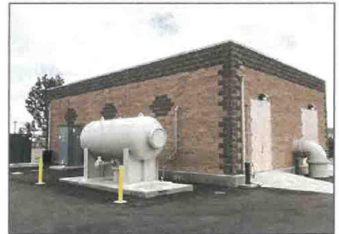
La Palma Water Complex City of Anaheim
