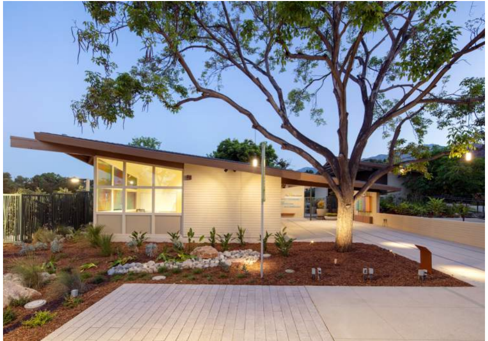
Rehabilitated Gate House - photo by SKA Studios
