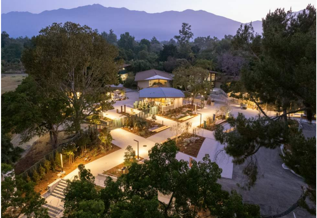
Los Angeles County Arboretum Entry Plazas & Gate House Rehabilitation Project completed June 2023
