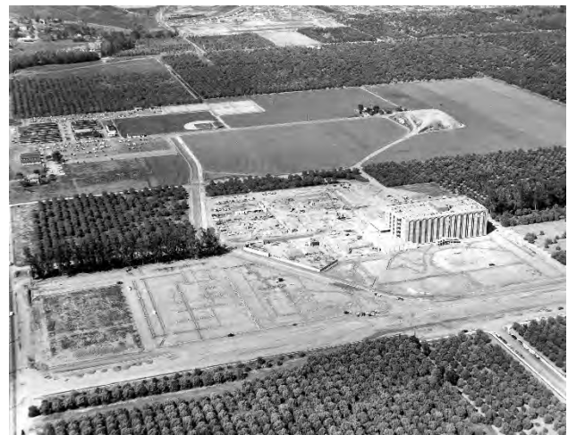
Cal State Fullerton under construction in 1963. Image from the Fullerton Public Library
