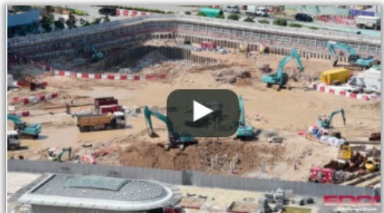
Construction & Demolition Processing Facility
