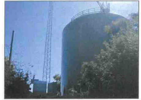
Wulff Tank Replacement Project Vallecitos Water District
