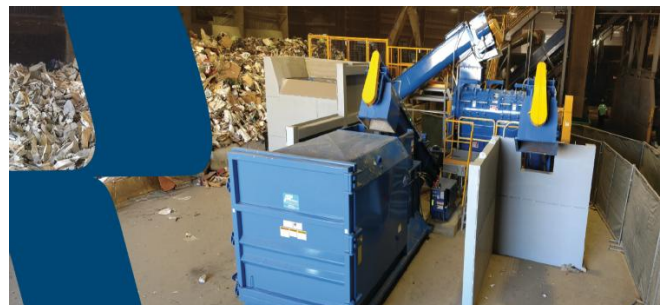
Figure 21. CVT . Republic Services New Recycling center Opened Spring of 2025 5 Miles away from Fullerton City Hall.
